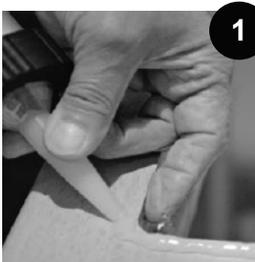
Cut out the countertop and apply silicone uniformly around edge.
